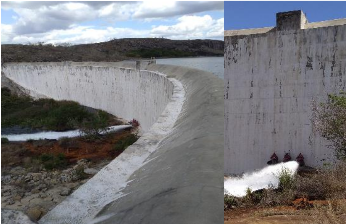
Photo 2.1 - Overview of Mugica Dam
