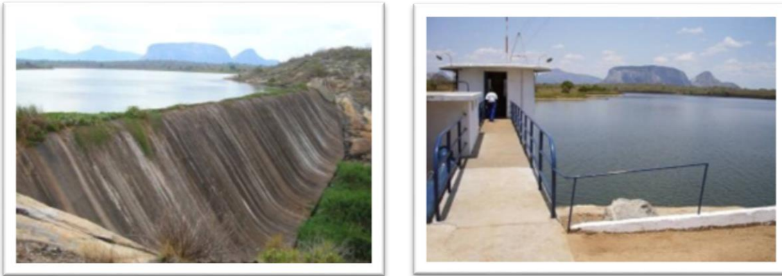
Photos 1 and 2 - Overview of Monapo Dam
